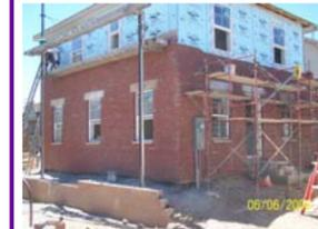
vendors such as Threewit Cooper Cement Co., Robinson Brick Co. and Rio Grande Co. We then put our unit masonry crew on the job and installed 8000 brick, 62 lf of stone sills and heads, washed, demobilized and turned it over to the painters and landscapers
